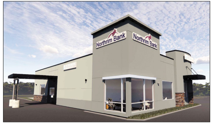
A rendering of Northrim Bank’s new Kodiak branch, which opened in February
